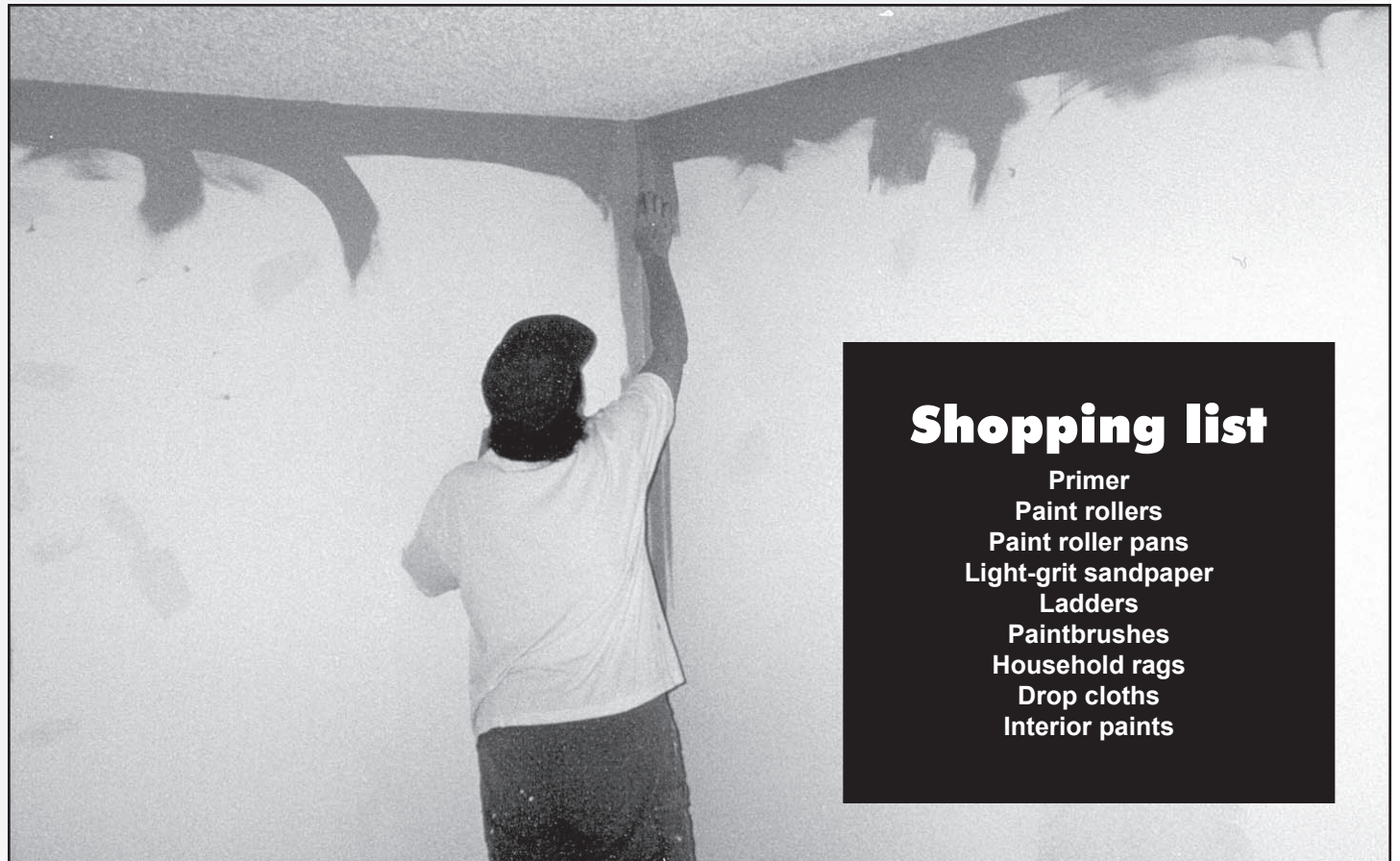
Using a special foam applicator helps apply an adequate paint coverage where the walls meet.
